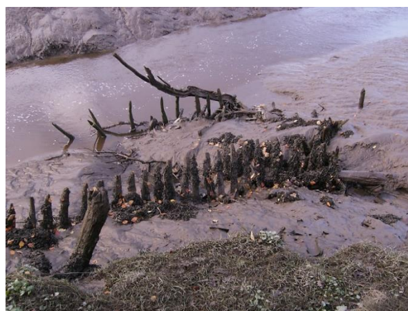
Figure 17. Seaward end of sluice box.
