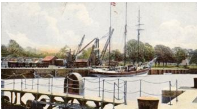
Figure 12. View of Alloa Wet Dock, circa 1903.
