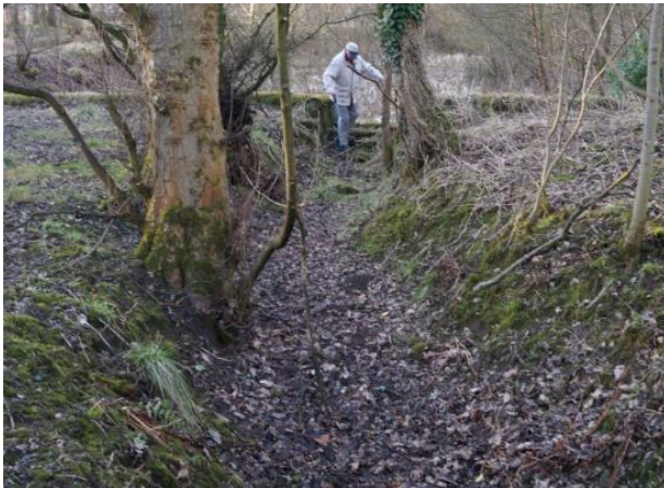
Figure 7. The pond dam overflow, 2015.
