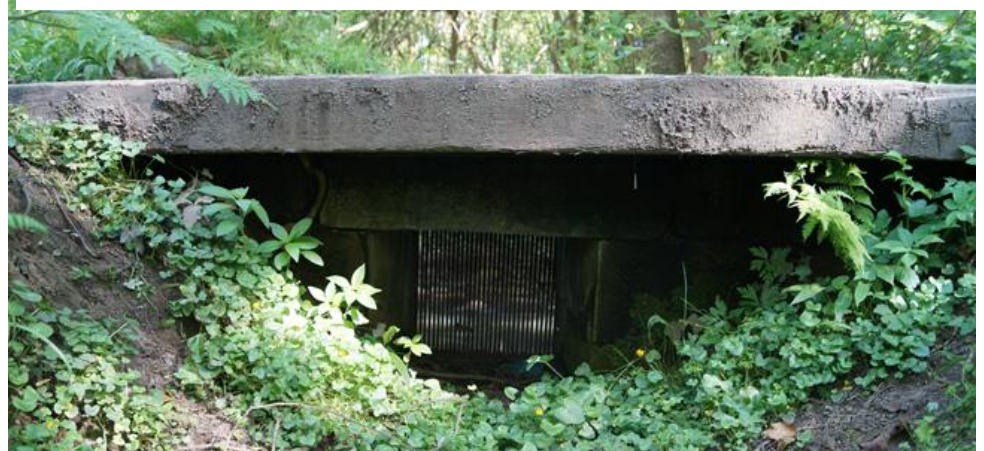
Figure 58. Inlet sluice, landward side.
