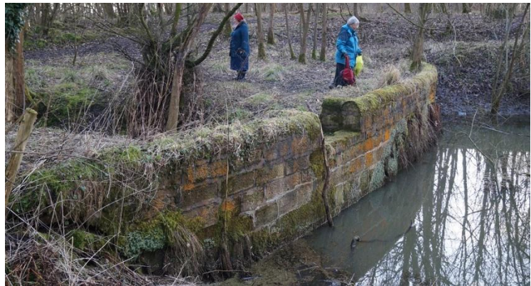
Figure 6. The pond dam, 2015.
