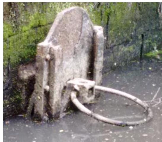
Figure 34. Front of the sluice.
