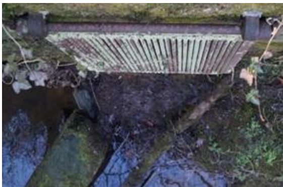
Figure 10. Metal grill at inlet sluice.
