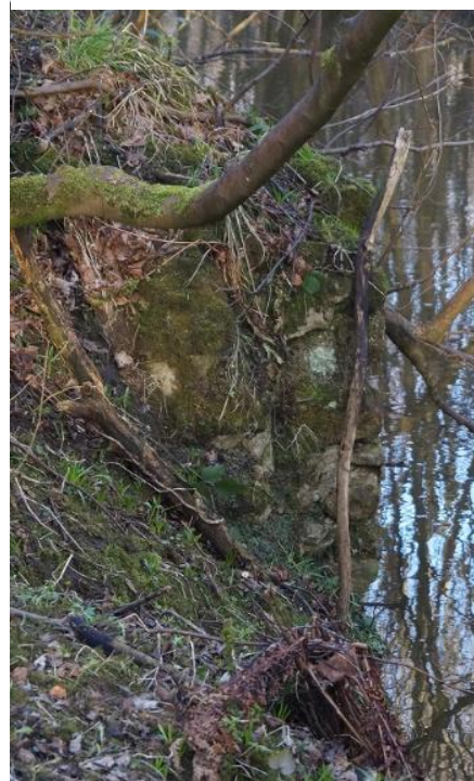
Figure 140. West bank end.
