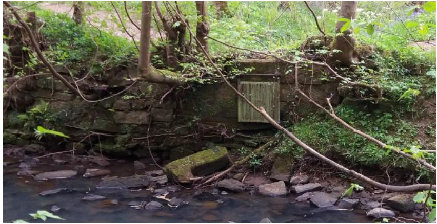
Figure 54. River side of inlet sluice.
