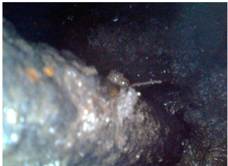
Figure 47. Metal rod in the base of the access pit.
