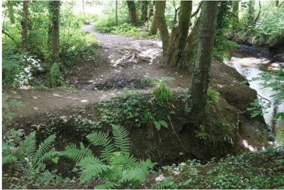
Figure 50. Overflow and culvert.
