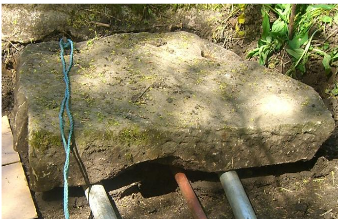
Figure 42. The access slab removed.
