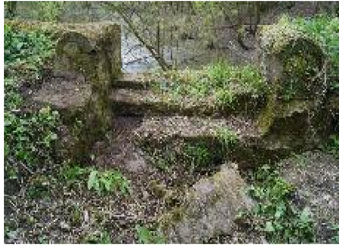
Figure 27. Overflow in the dam.
