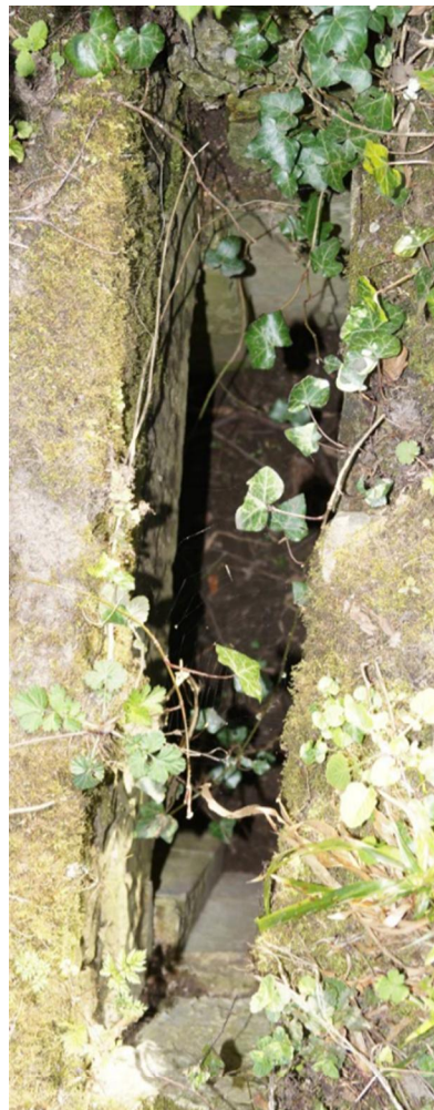
Figure 9. Niche for gate.
