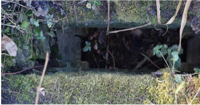
Figure 56. Inlet sluice gate guides.
