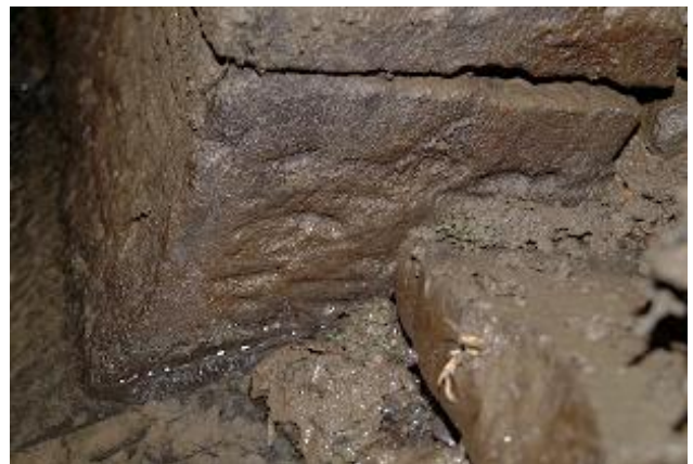
Figure 52. Cut stone arch.
