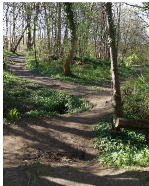
Figure 2. Path crosses culvert.
