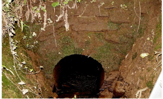
Figure 51. Drain enters culvert.
