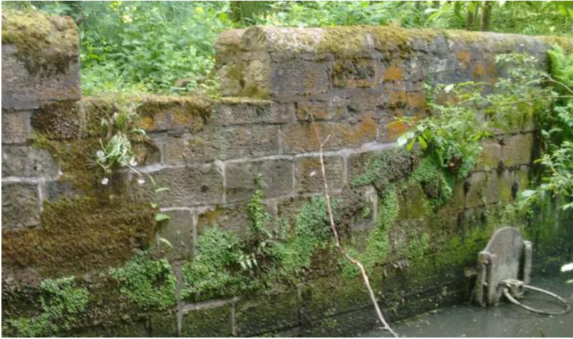
Figure 32. Overflow and drain location.
