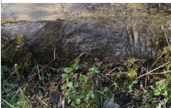
Figure 24. Rough coping stones.
