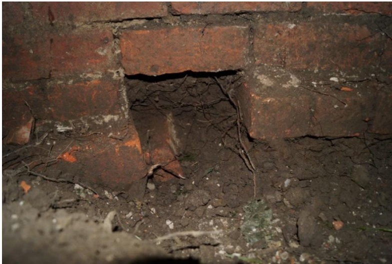
Figure 96. Ice house wall with stepped foundation.
