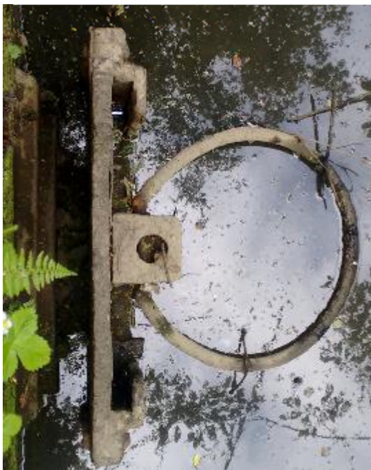
Figure 33. The sluice from above.
