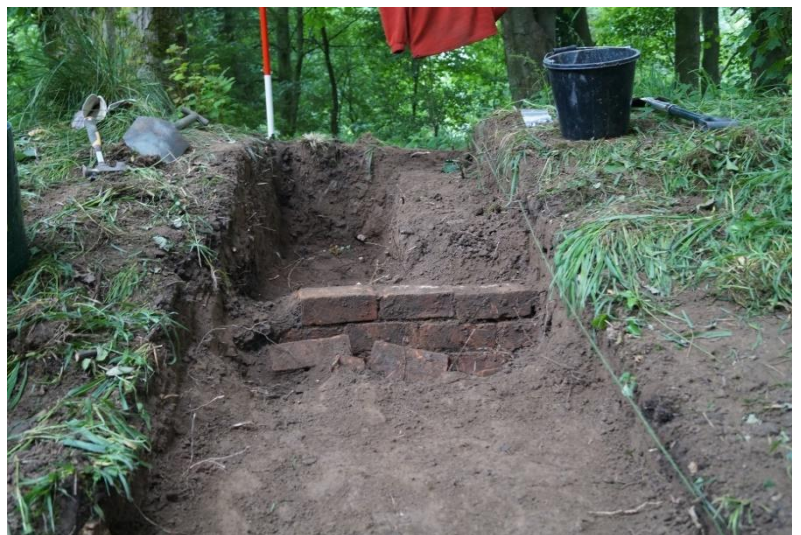
Figure 91. Ice house wall revealed in side trench.
