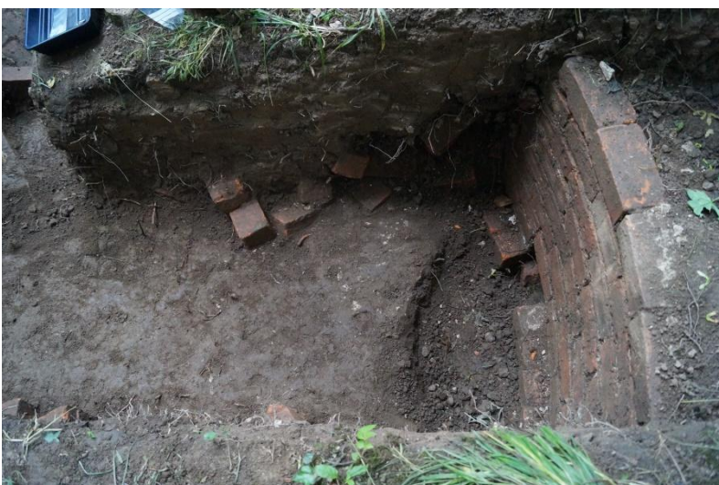
Figure 95. Ice house wall with foundation exposed.
