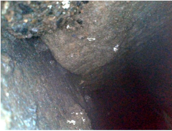
Figure 44. Blocks in access pit.
