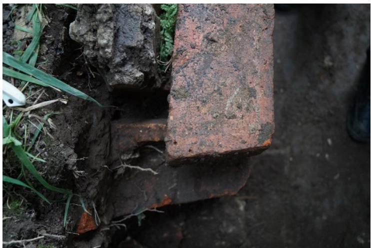
Figure 103. Cut brick at entrance.
