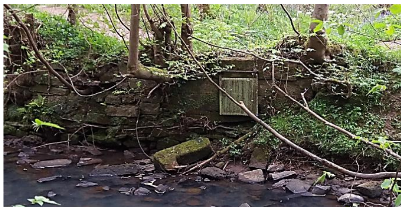
Figure 141. Inlet sluice built into older structure.
