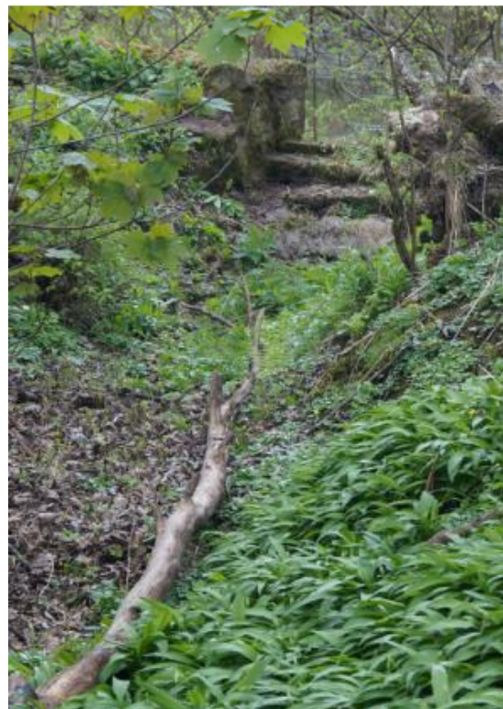
Figure 29. The overflow ditch.
