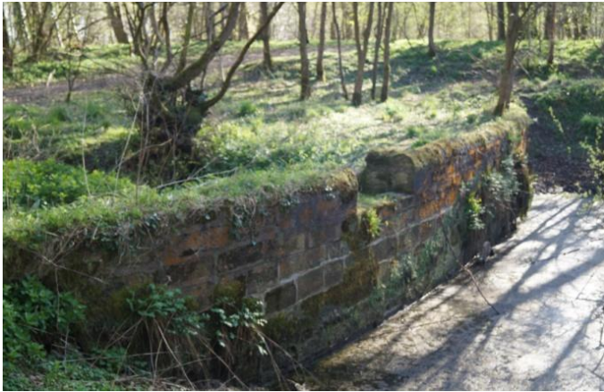
Figure 20. Arch shaped facing and overflow.
