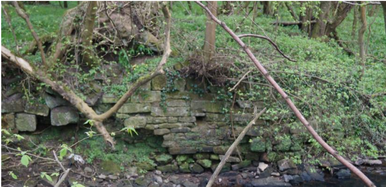
Figure 139. Possible remains of an early 18 th century or earlier bridge.
