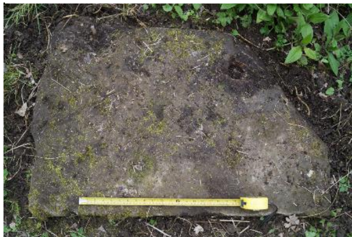
Figure 41. The drain valve access slab.
