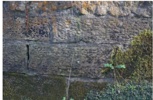
Figure 21. Well cut ashlar blocks.
