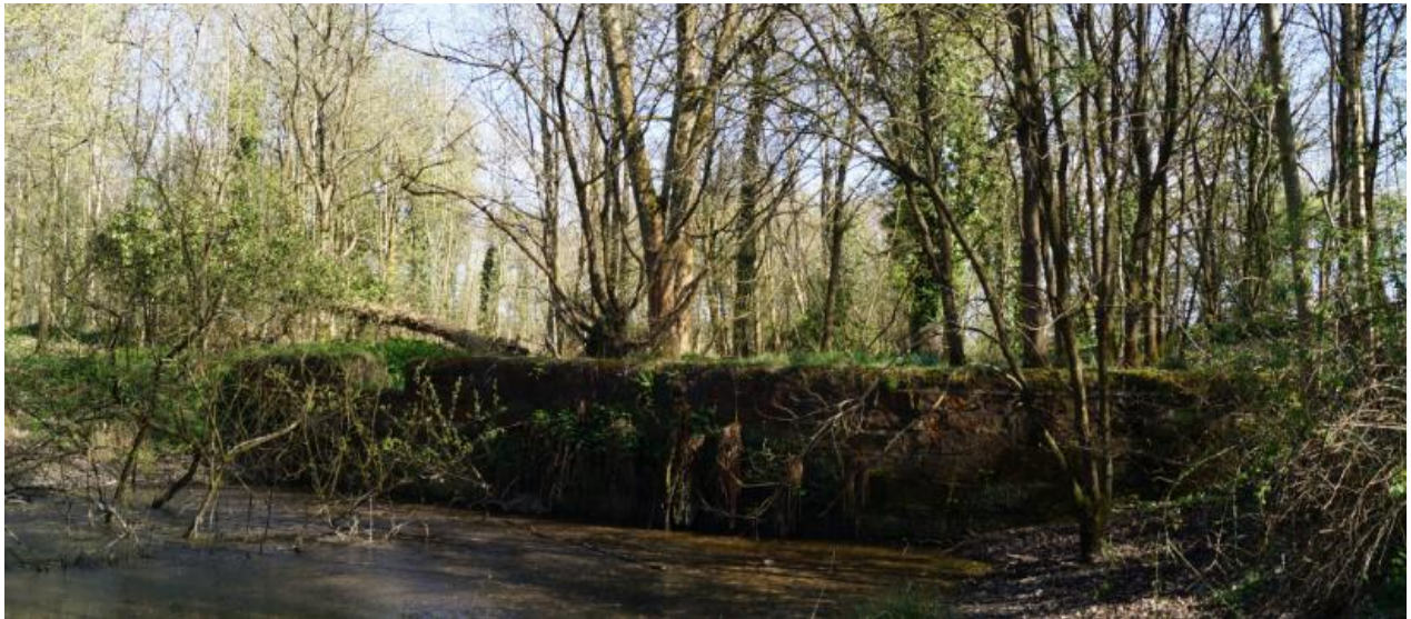
Figure 19. Sandstone facing to the earthen dam.
