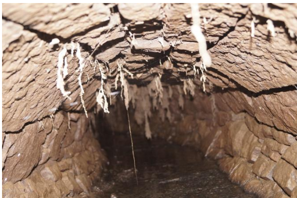
Figure 53. Roofed and floored drain.
