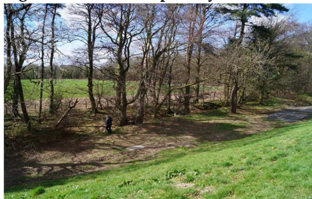
Figure 63. 1878 dam spillway ditch:
