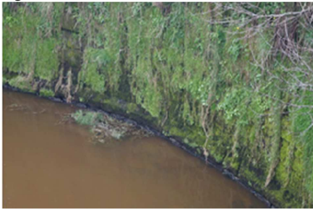
Figure 27. Two views of the stone kerb:
