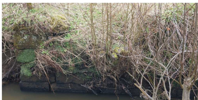
Figure 53. Stone culvert of Sauchie Burn.
