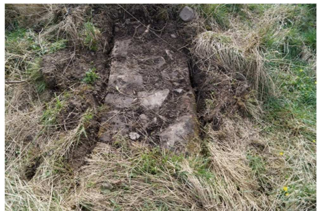
Figure 37. Wall from above.
