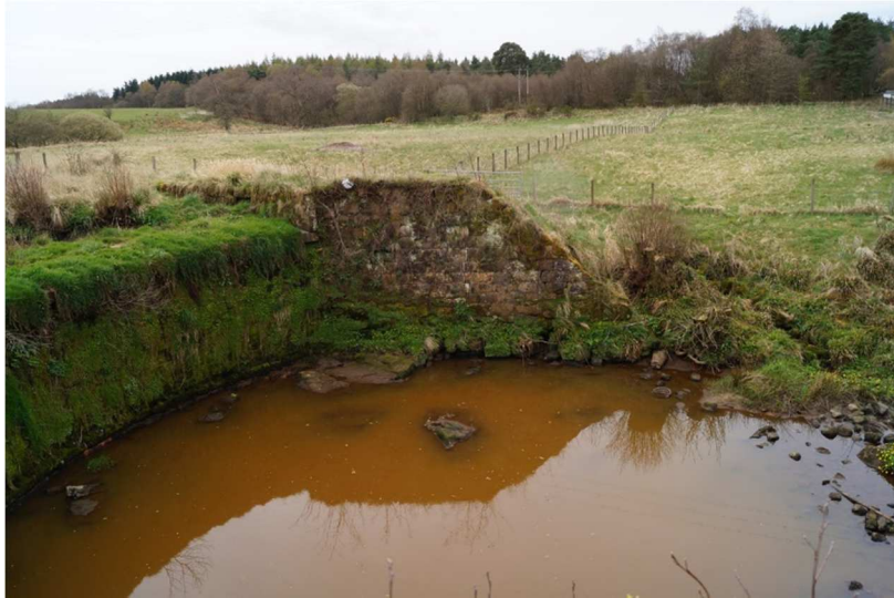
Figure 33. The southern buttress.
