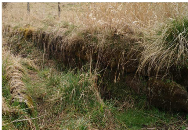
Figure 36. Rubble built wall.
