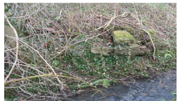
Figure 54. Remains of lade crossing.
