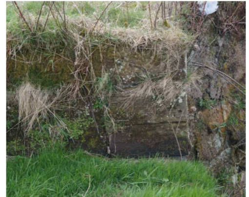
Figure 35. Weir edge of wall.
