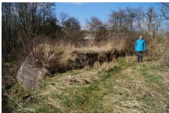
Figure 40. North buttress retaining wall.
