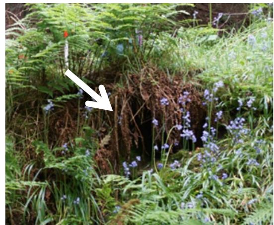
Figure 31. Location of pipe.
