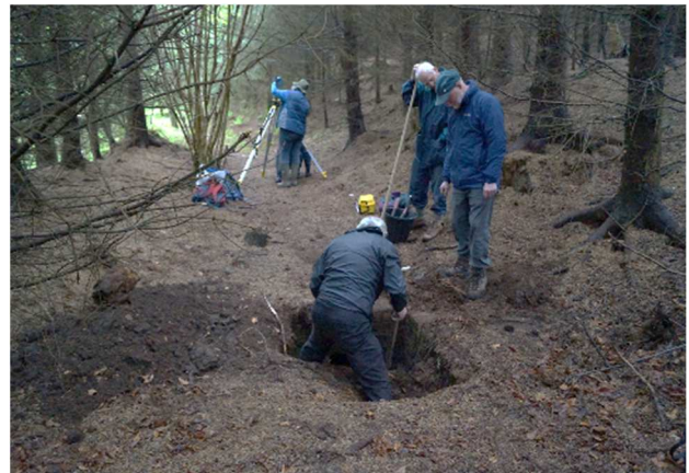
Figure 41. Excavation of manhole.
