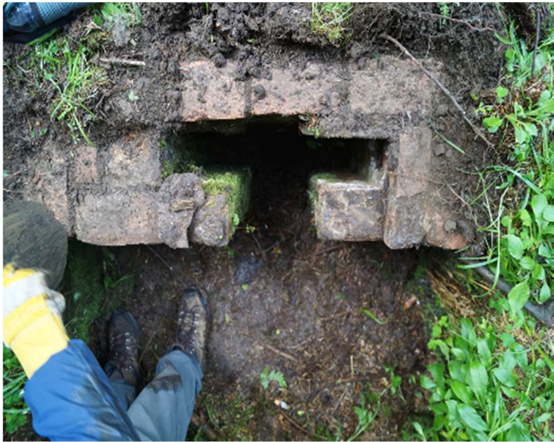
Figure 17. The drainage sluice area.
