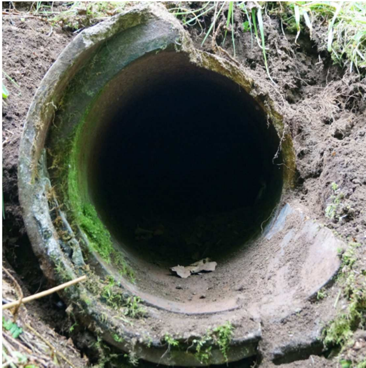
Figure 33. Faucet pipe end details.
