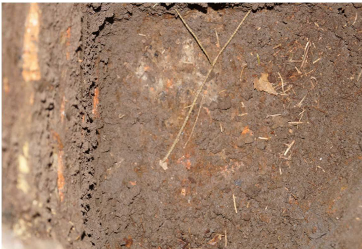
Figure 18. Lime and sand seal in sluice space.
