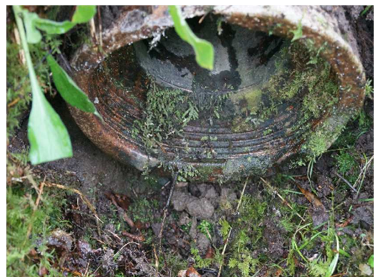
Figure 19. End of drain pipe.
