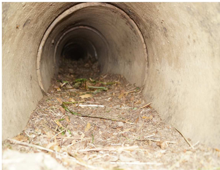
Figure 29. View up section of pipeline.
