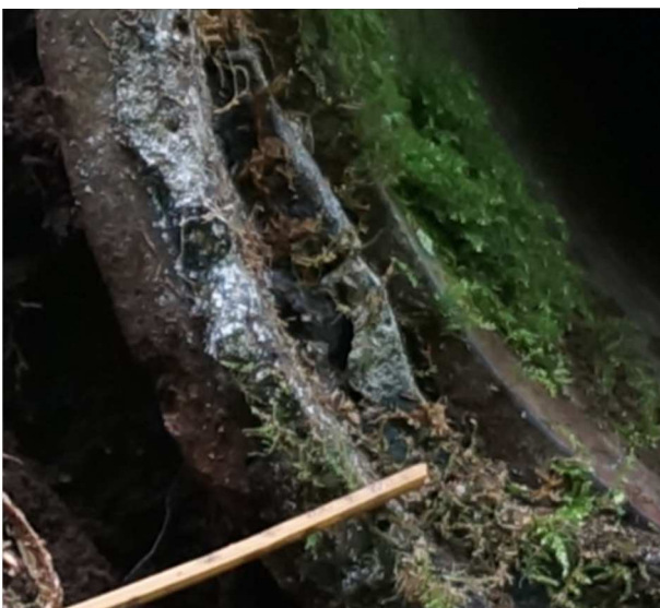
Figure 35. Detail of mortar seal.
