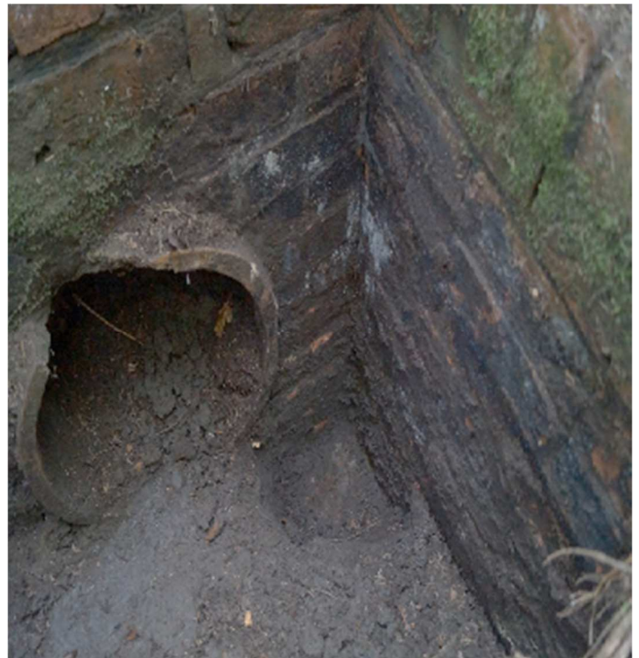
Figure 43. Inlet pipe and concrete base.
