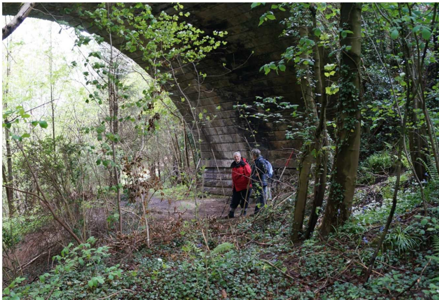
Figure 49. Lade passing under the railway viaduct.
