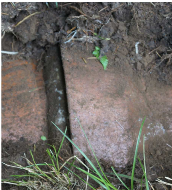
Figure 25. Detail of pipe joint.
