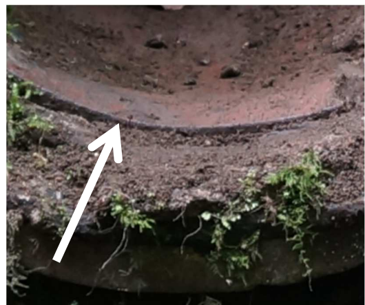
Figure 34. Faucet pipe end detail.
